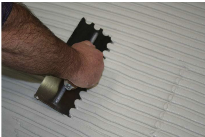
Picture 1.2 – 18 mm loop notch trowel with a medium bed mortar used for large format tiles or stones. Trowel thin set mortar in one direction holding trowel at a 45 degree angle. Notice the full ribbons of mortar that left behind.
